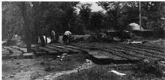
Bob Bosworth prepares to build first unit of his church and Bible school in Salisbury.
