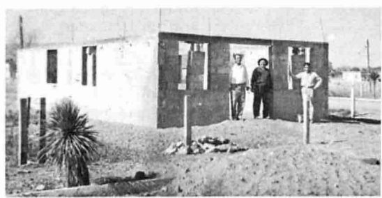
The church in Sabinas Hidalgo, Mexico, now ready for the roof of galvanized tin.
