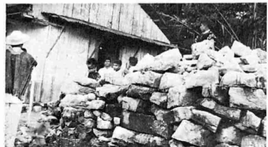
In front of the old wooden shack in which the Christians in Aguacatlan, Mexico, have been worshipping, are piled up the rocks with which they will build a new church.
