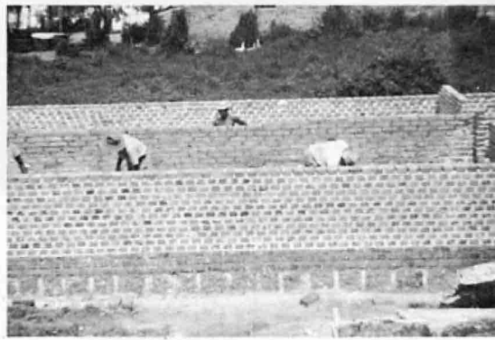
Some of the Christians at Encruzilhada do Sul, Brazil, erect the walls of their new church.
