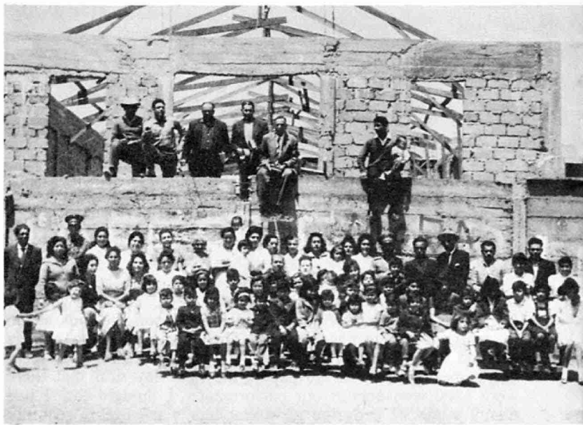
Church nears completion at Antofagasta.
