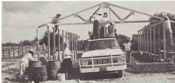
As building progresses, the kids become inspired and offer their help. Below: First truss goes up.
