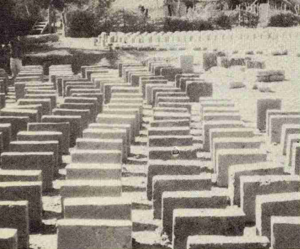
Above: Adobe bricks are made two miles away at the river. They are made of mud and set in the sun to dry. Below: Dirt is mixed with water to form mud used to hold adobe together. No cement is used except directly above windows and doors.
