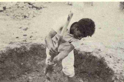
Above: Adobe bricks are made two miles away at the river. They are made of mud and set in the sun to dry. Below: Dirt is mixed with water to form mud used to hold adobe together. No cement is used except directly above windows and doors.
